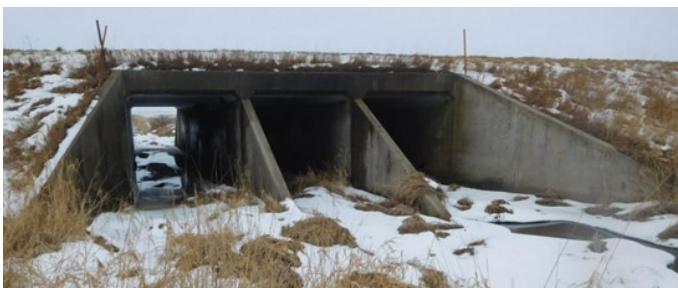
Concrete Box Culvert
