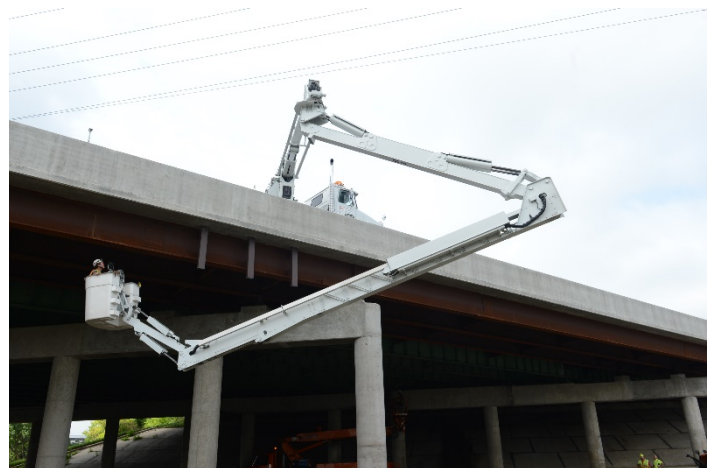
Under Bridge Inspection Vehicle
