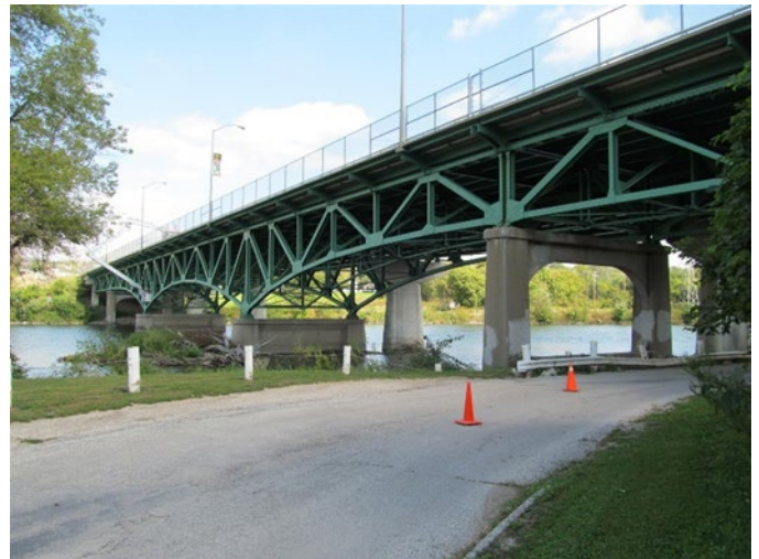
Steel Under Deck Truss
